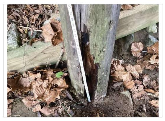
Bent 2 pile "D" decay
