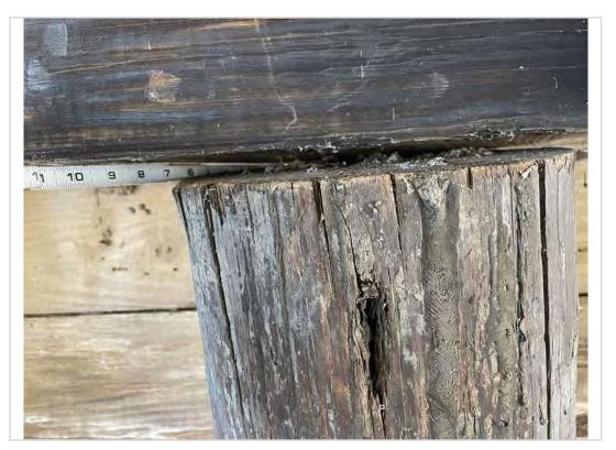
Abutment #1 pile E not fully contacting
